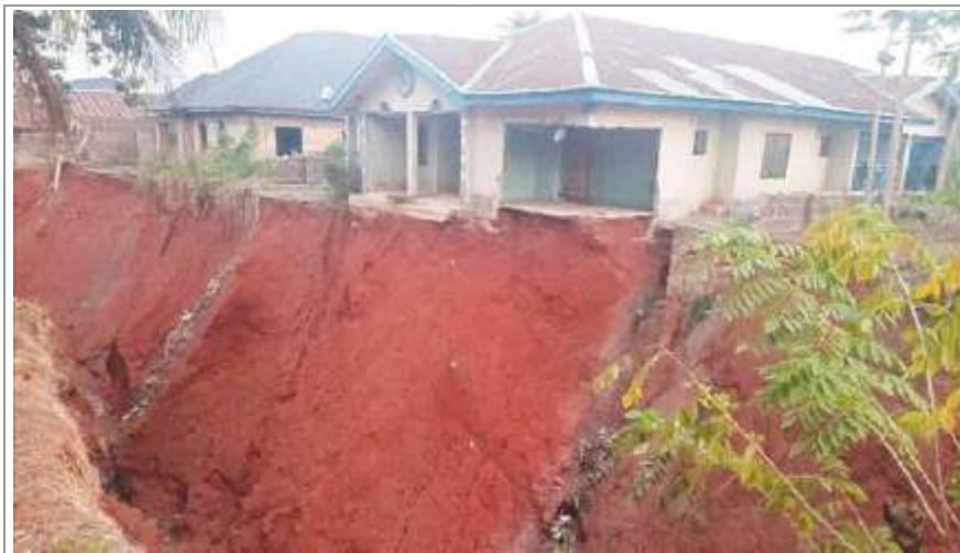
4.18: Erosion ravages Anambra communities (Source: Punch. December 21) 2023).
