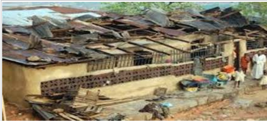
Figure 4.15: Windstorm destroyed shelters in Borno state
