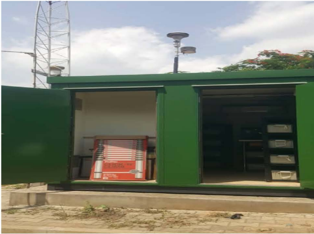
Figure 7.1: Exterior Abuja air quality station
