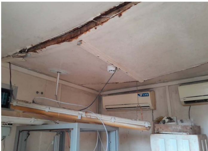
Figure 5.3: Dilapidated interior of Air Quality Station in Enugu
