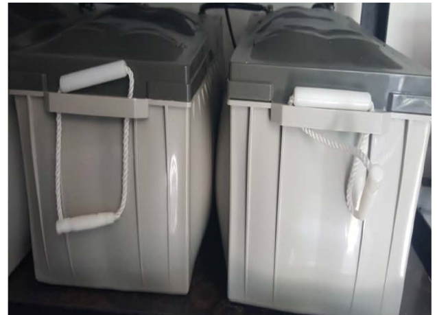
Figure 7.3 Swollen inverters batteries caused by exposure to high temperatures
