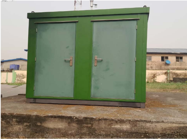
Figure 6.1: Exterior of the Lagos Air Quality station
